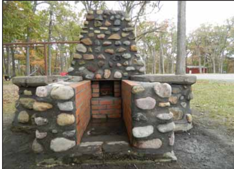
Renovated fireplace at Chautauqua Park
